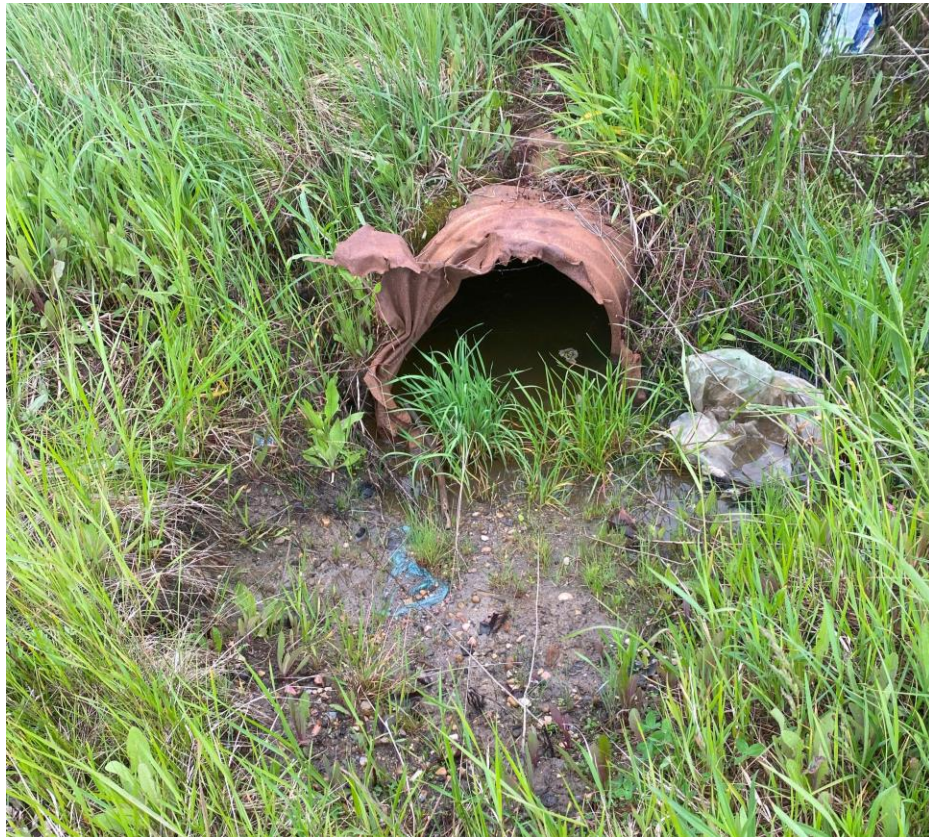
Figure C.4.-2: Partially buried and damaged through-grate culvert at Hwy 626 near the intersection with 47 St.
