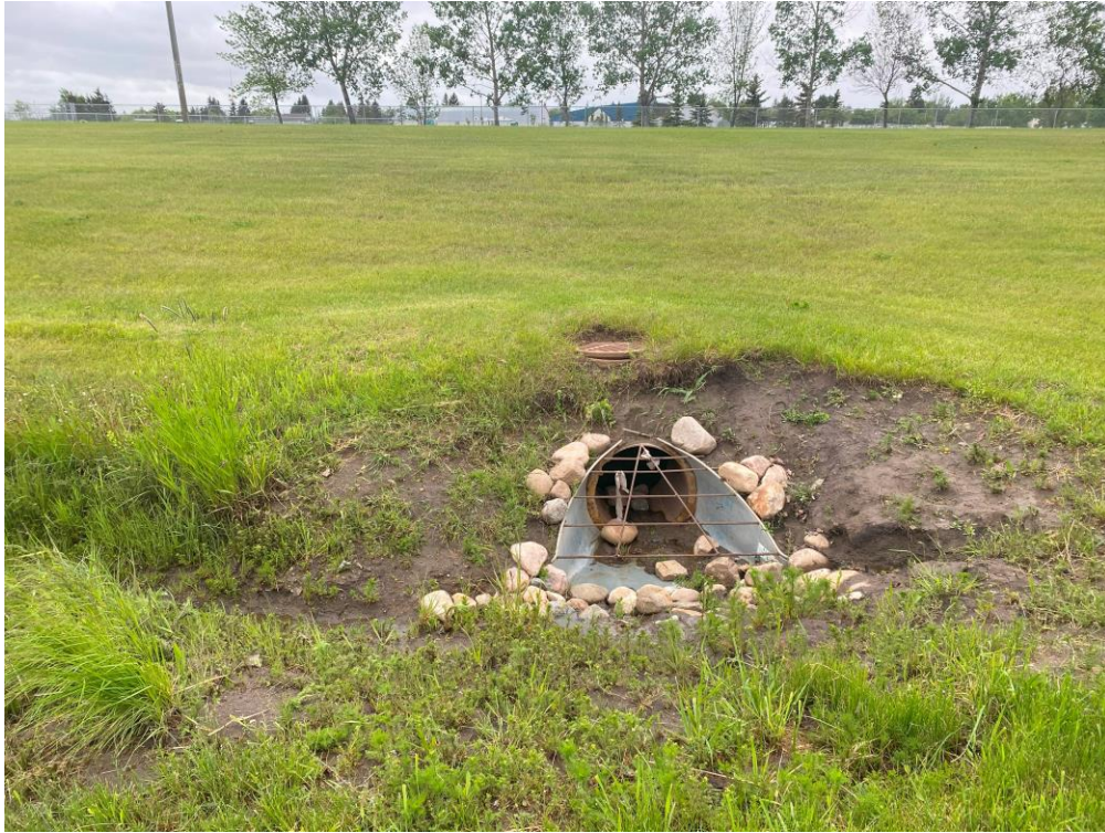
Figure C.4.-5: Storm sewer inlet along the 47 St east ditch – looking west.
