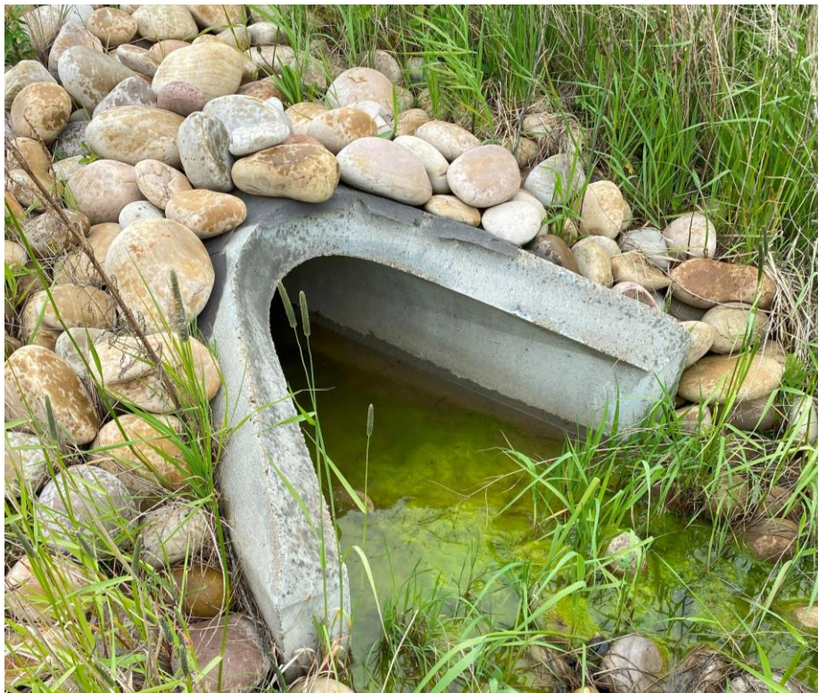
Figure C.4.-12: Manhole overflow pipe outlet near the lift station.
